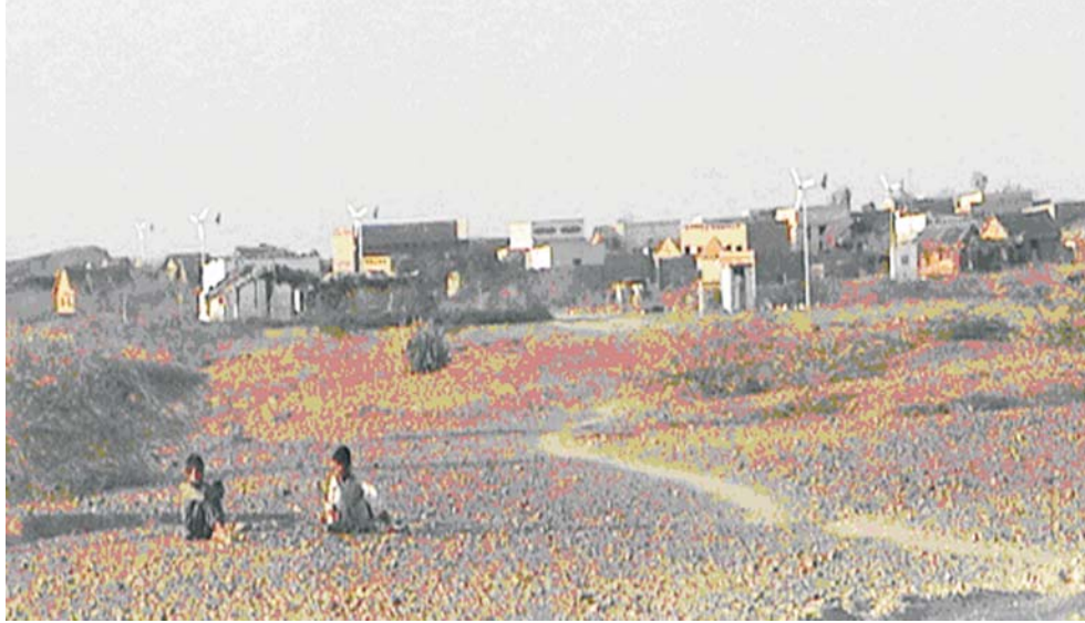
Figure - 1: A Panoramic View of the Village Gul Muhammad, 1st Pakistani Village Electrified by PCRET using Wind-Energy
